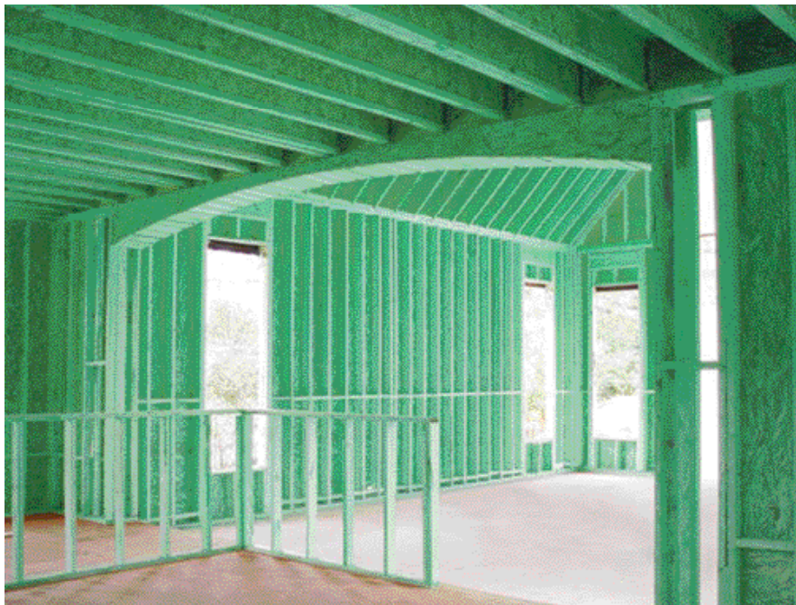
Factory-applied treatments like FrameGuard (shown here) protect against mold, decay, and insects.
